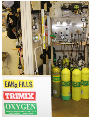
8 tank whip fill panel with O2 clean mixing block & panel O2 regulator
